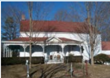
The historic c.1730/1760 Lester house (later Weiland) in Clinton Corners
