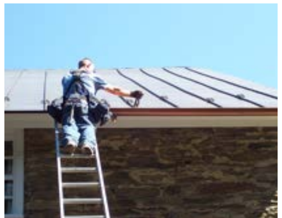
The roofer shown installing our new copper roof.
